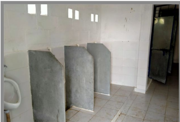
Construction of sanitation blocks for boys in Choranda and Handod Schools at Karjan
